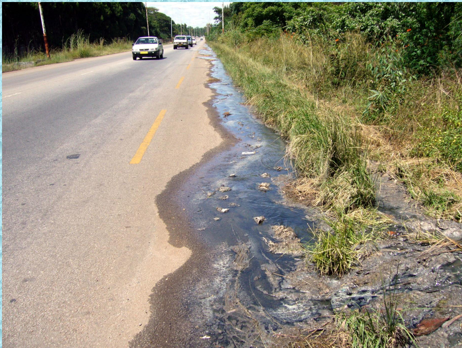
Breached sewer effluent flowing along suburban road in a middle to high income area
