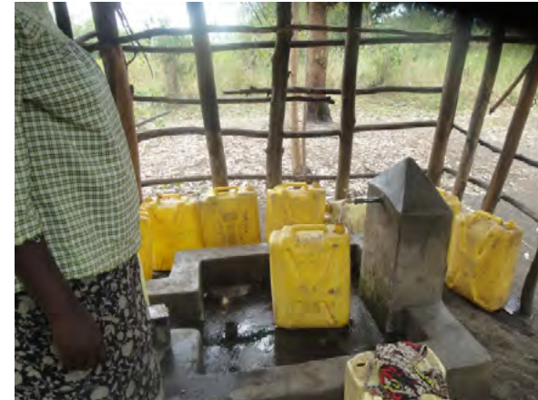
Figure 6 - Water collection at standpipe from a gravity scheme
