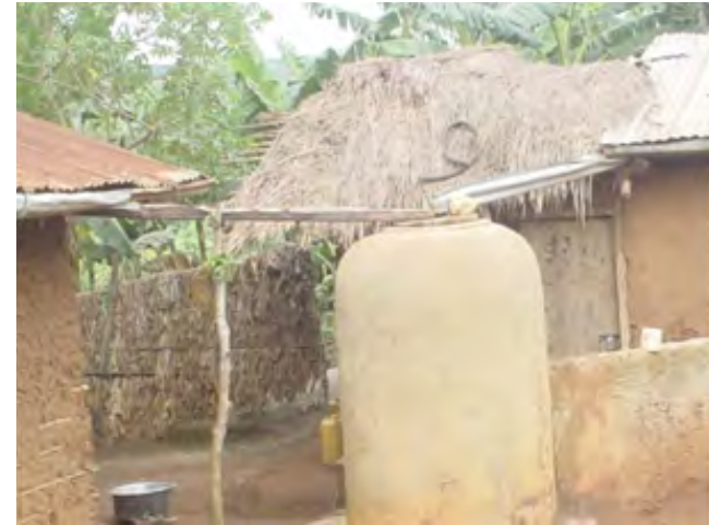
Figure 2 - a ferrocement rainwater tank
